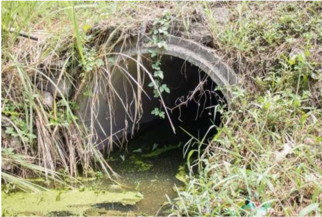
Figure 1.1- Drainage through pipes
