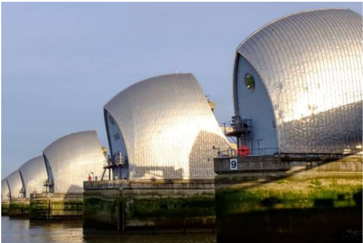
Figure 9 Thames Barrier which protects London from tidal flooding. Rising sea levels will mean the Barrier is closed more frequently.
